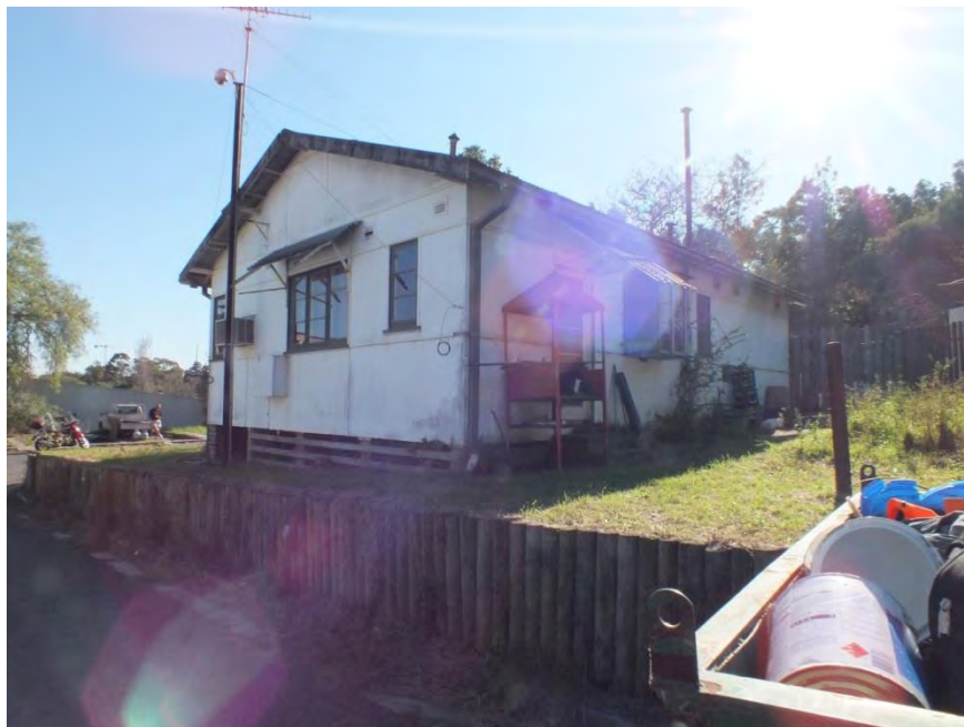
Figure 3.10 View northwest of post-1930s fibro dwelling, constructed on brick piers on terraced embankment (Source: AM Consulting).
