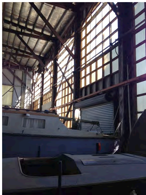
Figure 6.02. Original Building, Original Timber Glazing Framing, Looking West
