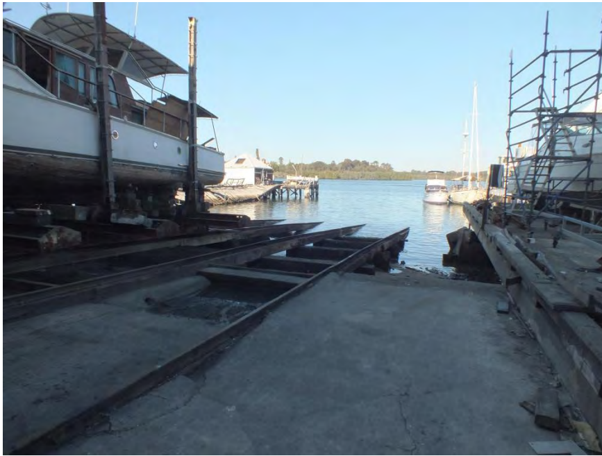
Figure 3.5 View southeast of two remnant Halvorsen's slipways and partially collapsed wharf (Source: AM Consulting).
