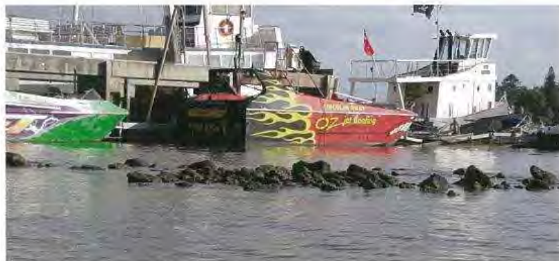
Figure 10. Foundation remains of James Squire's wharf exposed at low water springs, January 2014. These sandstone blocks are in the same position as the trace of the wharf visible in Figures 8 and 9.
