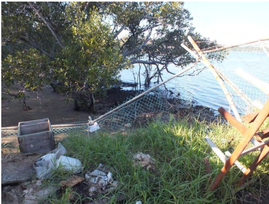
Figure 3.6 Recolonised mangroves and refuse lining the foreshore to the east of the main warehouse (Source: AM Consulting).
