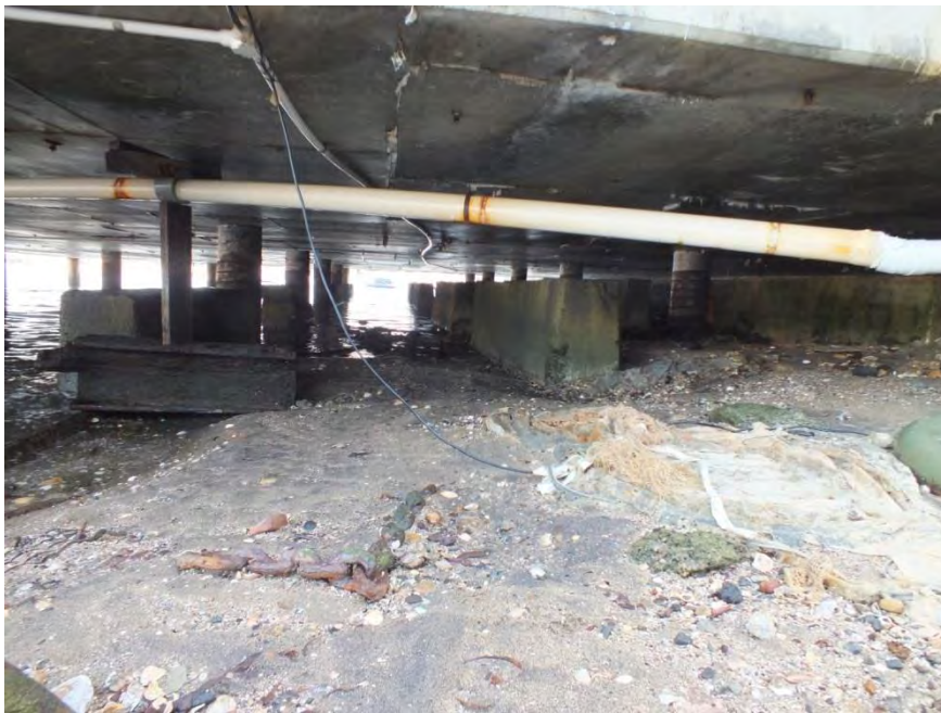
Figure 3.4 View west of the foreshore and concrete pylons beneath the concrete apron. Note the tidal wash-in of shell, netting, fibro fragments and general debris (Source: AM Consulting).
