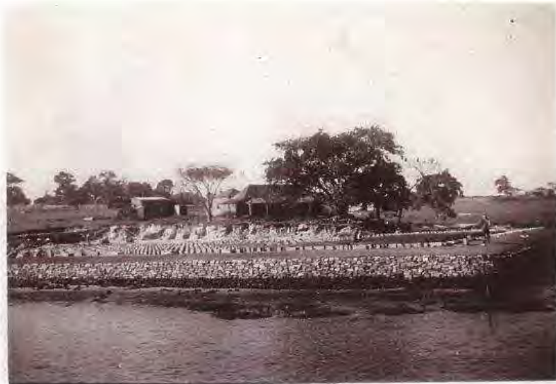
Figure 5 Construction of Halvorsens boatshed circa 1939/40. Sandstone was excavated to provide a level foundation and dressed blocks were placed in the seawall. The original house and outbuildings in the rear were demolished soon after this photo was taken. Note that the depth of the foundation cut at the rear of the building is probably sufficient to destroy any original building footings. Photo from Randi Svensen collection held by the National Maritime Museum, Darling Harbour.
