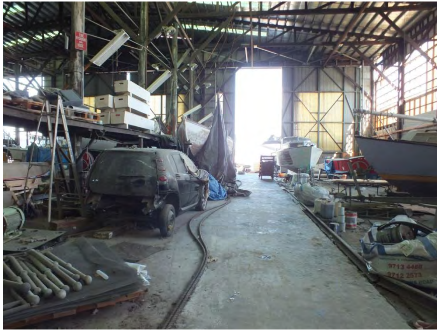
Figure 3.11 View along the western 'aisle' to the south. To the left is the elevated working platform and to right the flooring is timber board, and note the slip rail (Source: AM Consulting).
